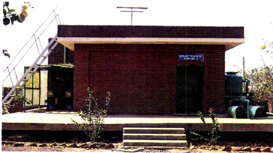
Sewage Treatment Plants (STP) at the campus
